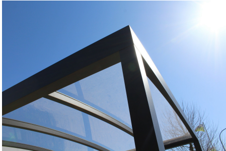
Transparent: 80-90% transmission de lumière
